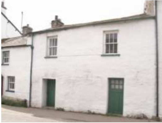
Low window to wall ratio Buildings built on pavement line (central village)
