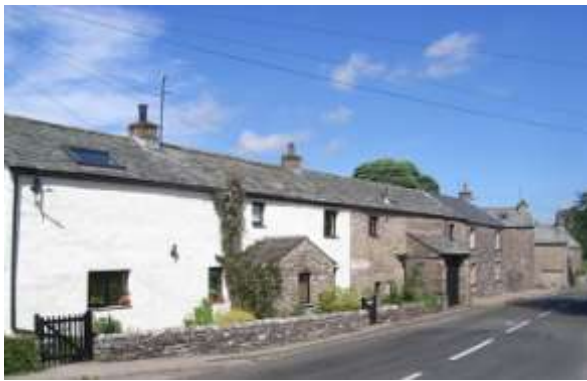
Former farmhouses with attached barns under one continuous roof Low limestone boundary walls Gable roofs
