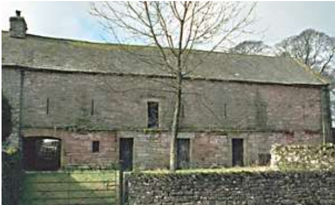
Barn and Byre Range Adjoining North End Of Petty Hall - Grade II
