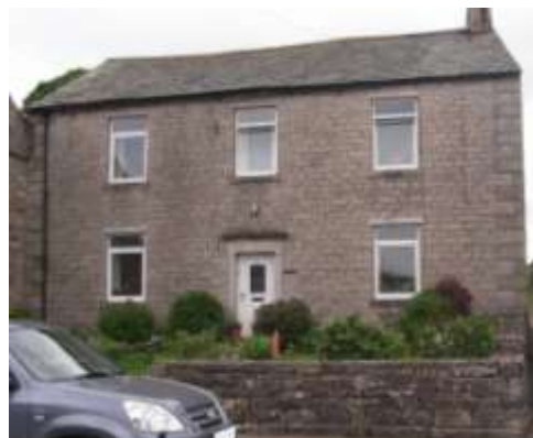
Modern casement windows
